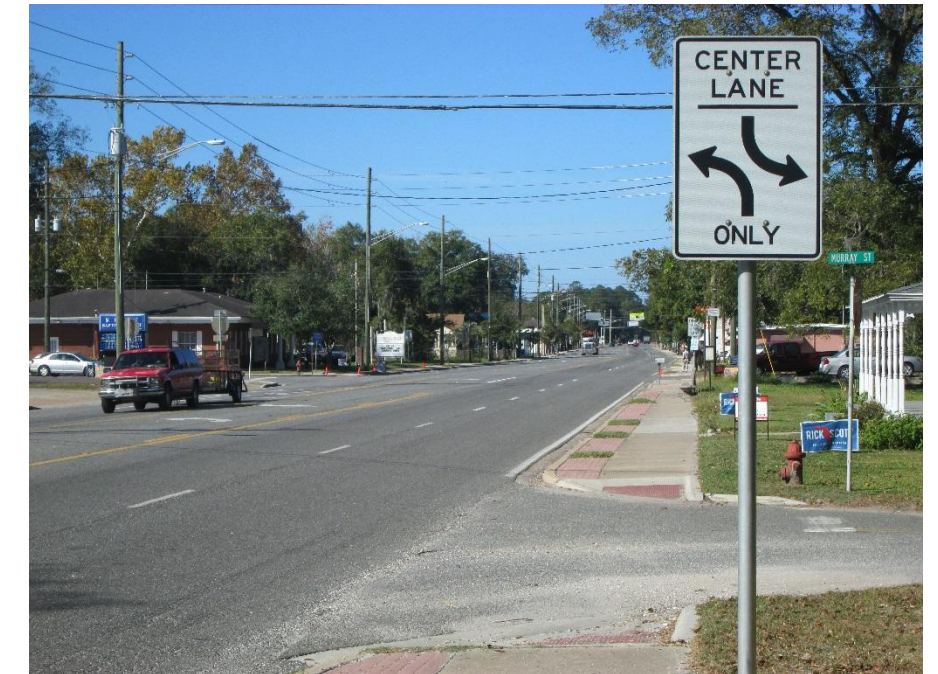
Access Management Issue – Existing Two-Way Left-Turn Lane in Baldwin, FL
