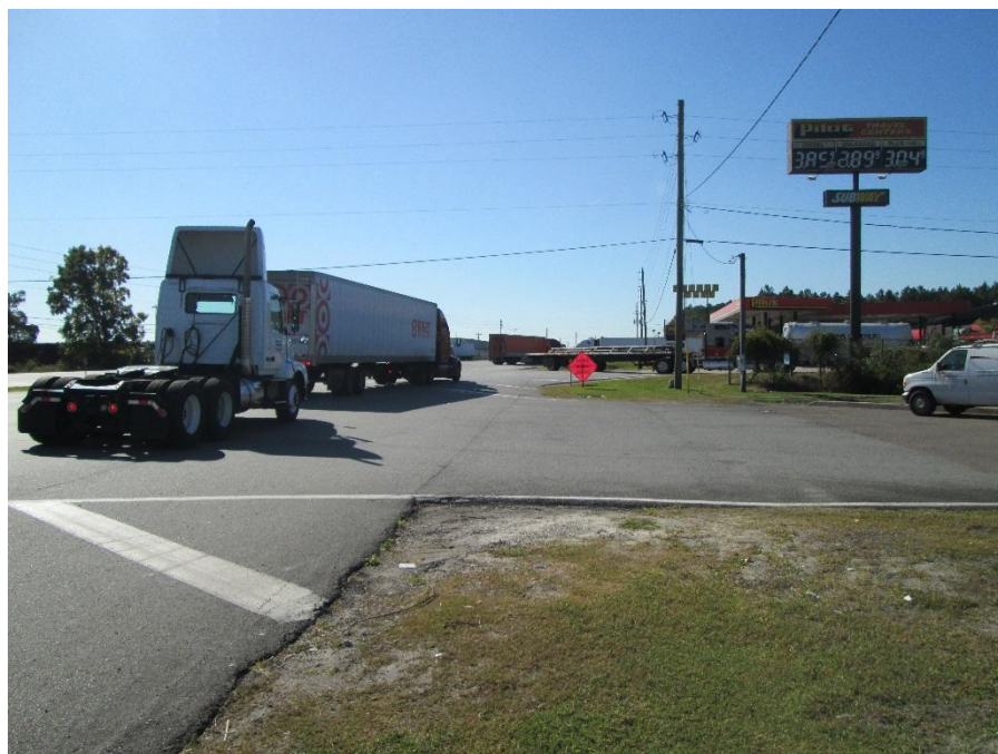
Inadequate Intersection Design, Starke, Florida
