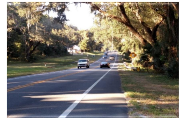
Two-lane roadway south of Belleview toward The Villages
